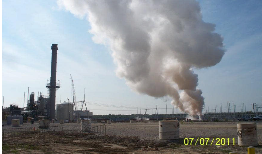
Unit 1 Steam Blow
