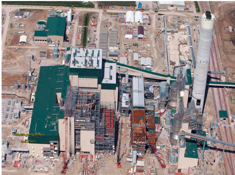
Power Block Construction
